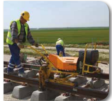
Robel FASTCLIP installation machine
