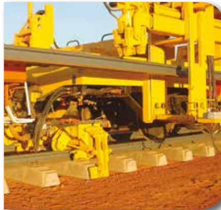
Harsco Track Laying Machine with integral clipping head.
